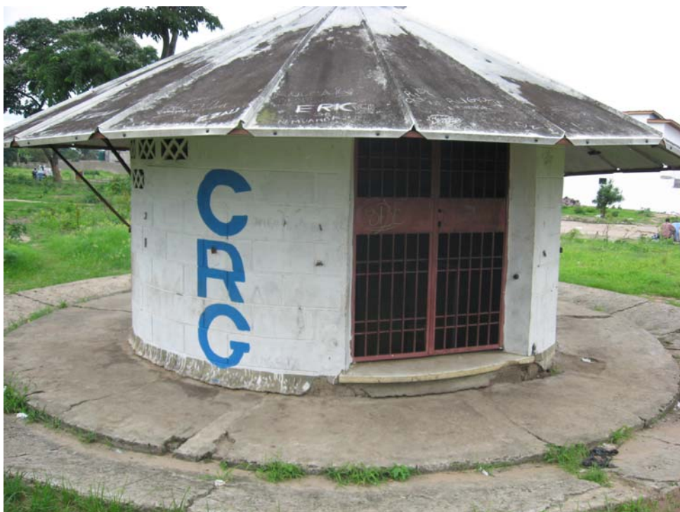
Fig1.: Outside view of Binza magnetic vault entrance.
