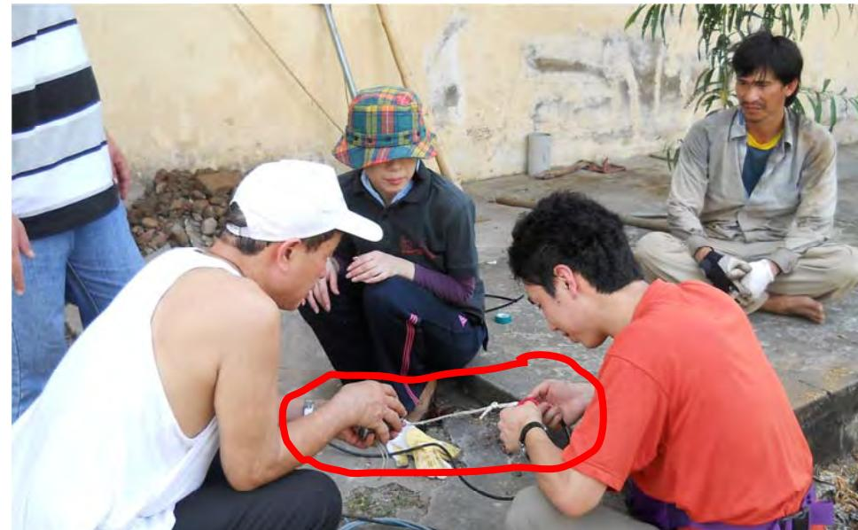
Pulling sensor cable through buried tube.
