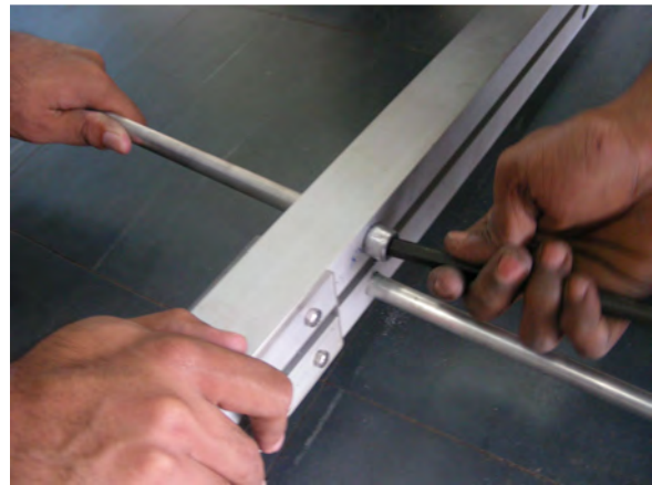
Fig. 2 Attaching the dipoles to the two booms. The two booms separate by 33mm using Perspex sheets.
