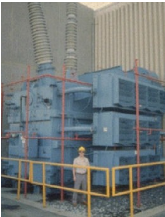
Permanent damage to the Salem New Jersey Nuclear Plant GSU Transformer caused by the severe geomagnetic storm of 13 March 1989 (Photos courtesy of PSE&G)
