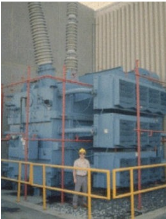
Permanent damage to the Salem New Jersey Nuclear Plant GSU Transformer caused by the severe geomagnetic storm of 13 March 1989 (Photos courtesy of PSE&G)
