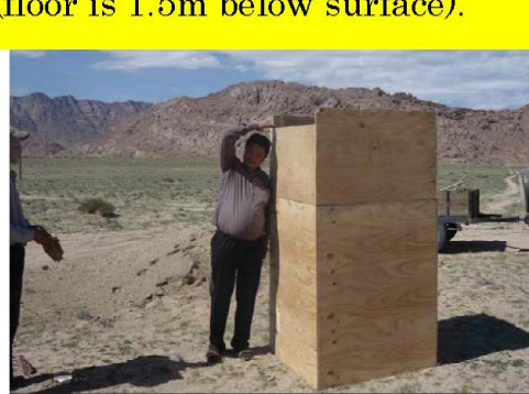
Construction of sensor house (floor is 1.5m below surface).
