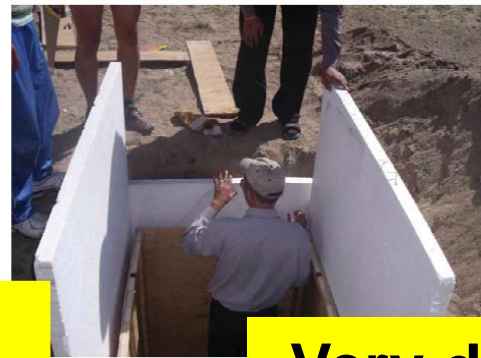
Construction of sensor house (floor is 1.5m below surface).
