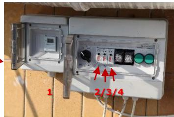
Controllers for the morning start time (1), time interval of one single rotation (2), duration of single antenna rotation (3), and evening stop time (4).
